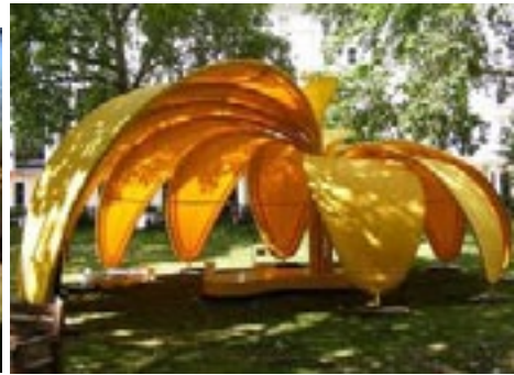
Fabric Tensile Structure
