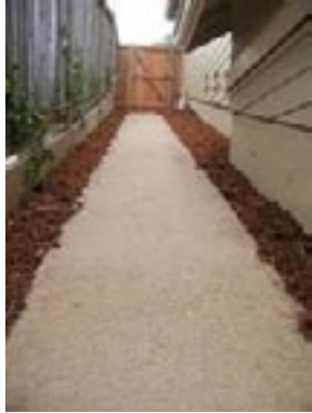
Loose DG walkway
