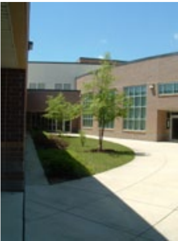
William Hall Elementary School Prince George's County Public Schools
