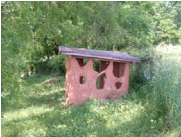
Handmade cob structure
