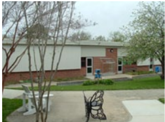
Brick masonry and metal siding
