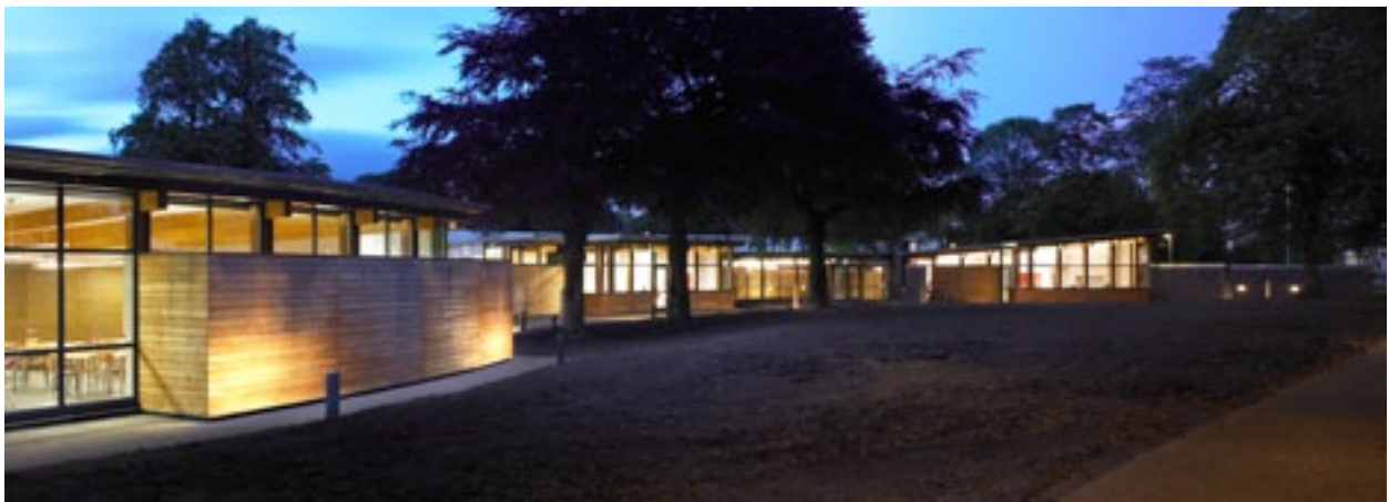
Wood siding and glazing
