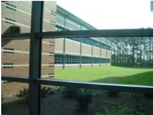
Brick masonry and ribbon windows
