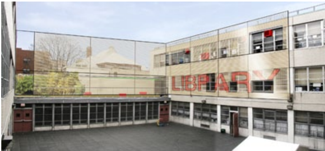
Supergraphics can add a fresh new feeling to an older building.
