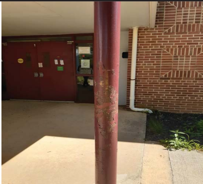
Picture 3: Exterior Red Metal Pole
