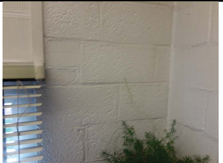
Picture 4: White CMU Wall
