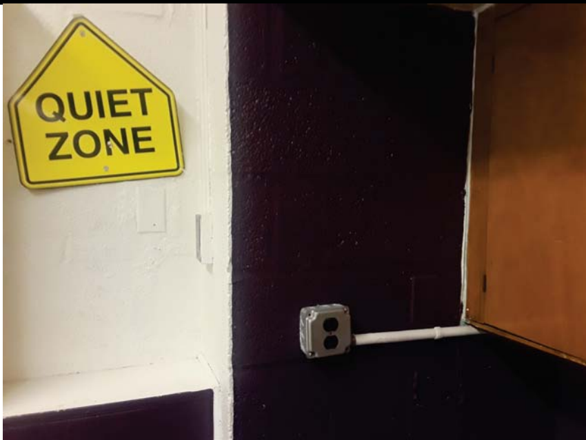
Picture 3: Purple CMU Wall
