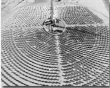
Photo credit: U.S. Department of Energy
