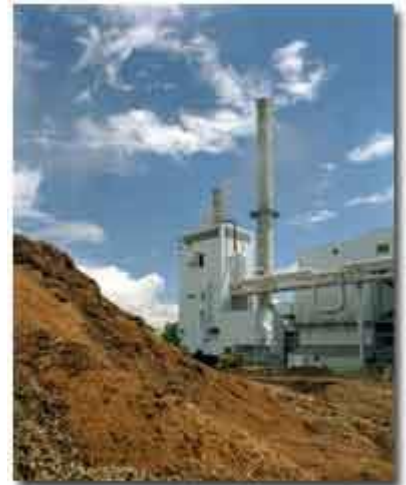
Biomass Power Plant - Photo credit: U.S. Department of Energy, Energy Efficiency & Renewable Energy Network (EREN)
