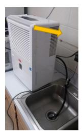
5. For dehumidifilers that drain continuously (in a sink, through a wall or into a condensate drain), check the drainage hose regularly to make sure there is flow and that the hose is sloped downward.
