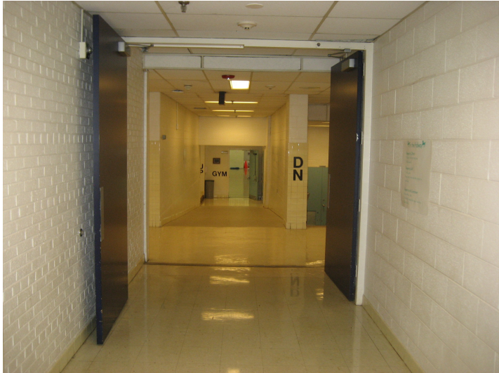
Corridor Ramp to Gym
