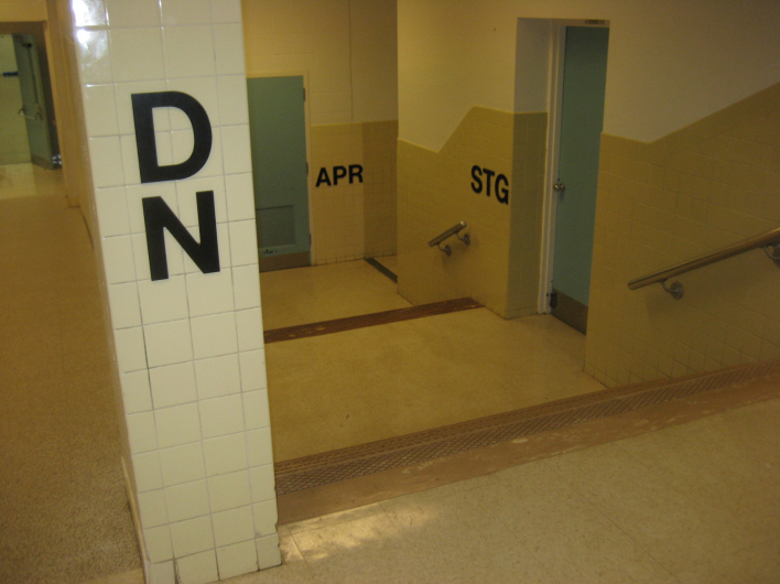
Stairs to Multi-Purpose Room
