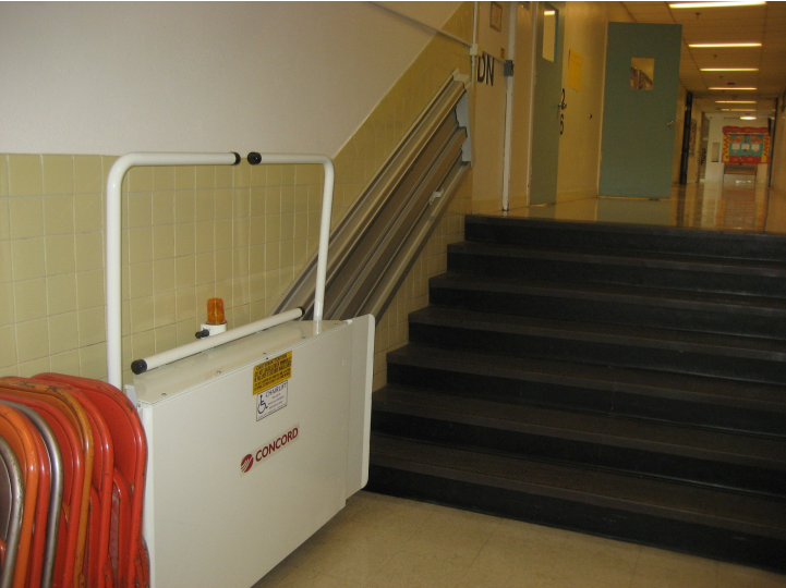
Stairs and Lift to Multi-Purpose Room
