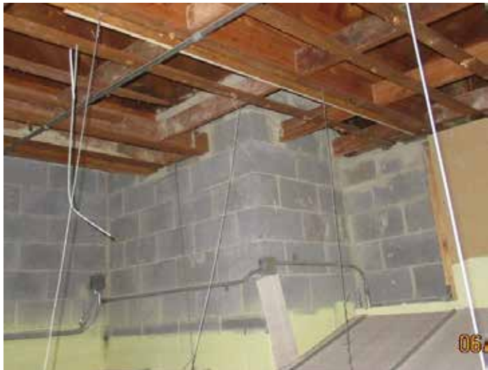
Glulam Wood Beams Over Current Pre-K
