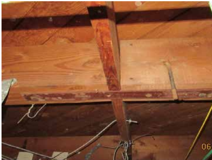
Connection of Cantilevered Beams at Corridor - 1952
