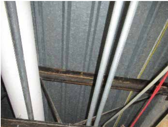
Joists and Metal Deck on CMU Walls
