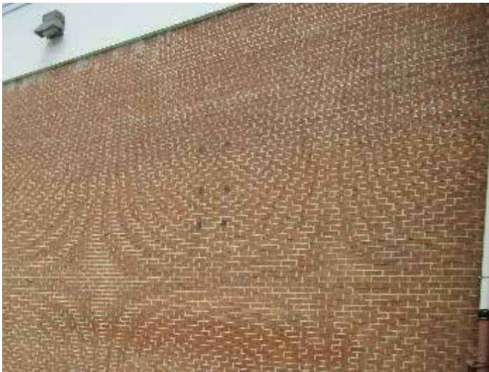
Exterior Gym Wall with Steel Plates and Rods
