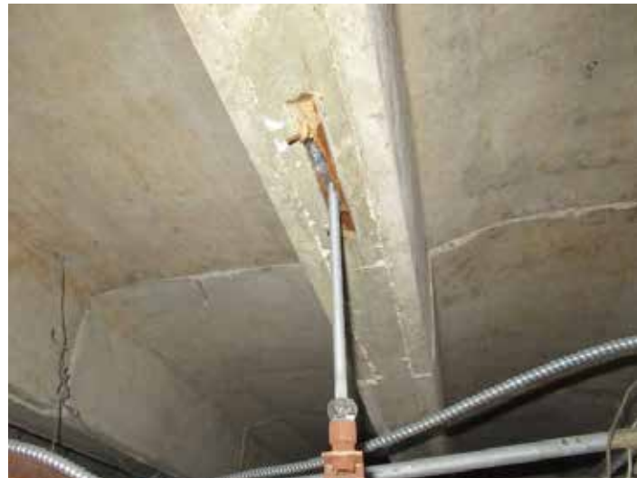
Existing Concrete Pan Joist Floor - 1959
