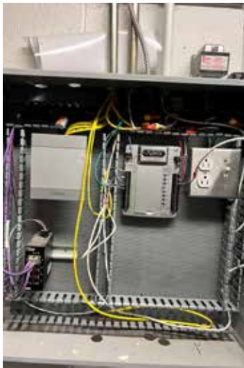
Existing ATC (automatic temperature control)
