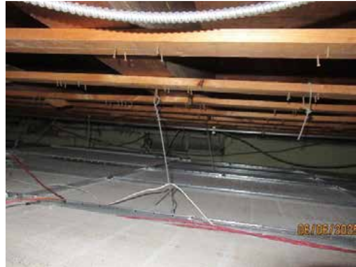
Built-up Wood Beam and T&G Roof Sheathing - 1955
