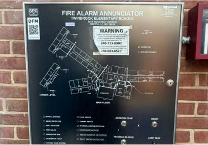
A fire alarm annunciator panel (FAAP) is located in the main entrance vestibule. Fire alarm devices include manual pull stations, smoke detectors, and audible and visual notification devices.
