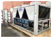
FIGURE 21. AIR COOLED CHILLER #2
