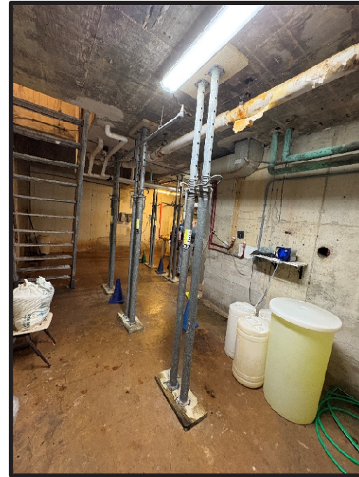
Figure 2 Prop columns below pool deck.
