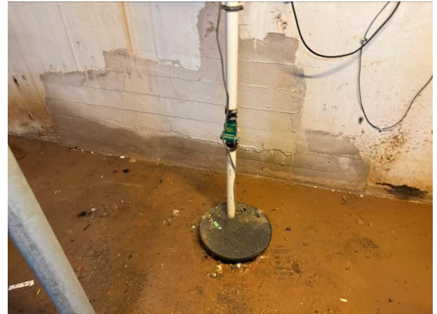
Photo #18 View of pool equipment room sump and drain system.
