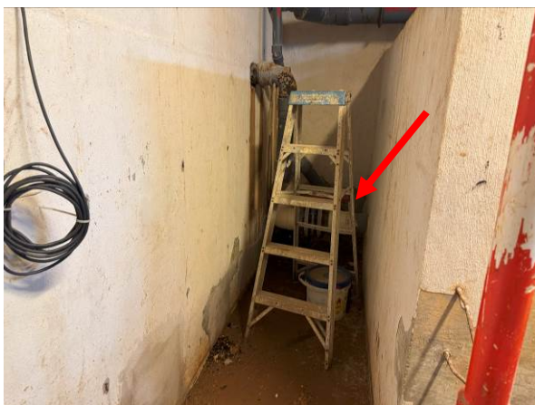
Photo #23 View of pool main drain piping into surge tank.
