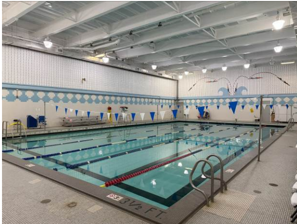
Photo #1 View of pool from shallow end entry onto pool deck from locker rooms and deck drains.
