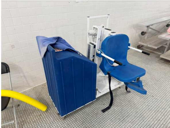
Photo #7 View of pool ADA access lift and tip and roll bleacher.
