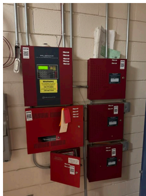
Fire Alarm Control Panel and Voice Control Panel
