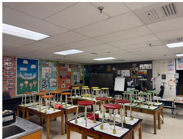
Typical Classroom Lighting
