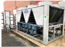
FIGURE 21. AIR COOLED CHILLER #2
