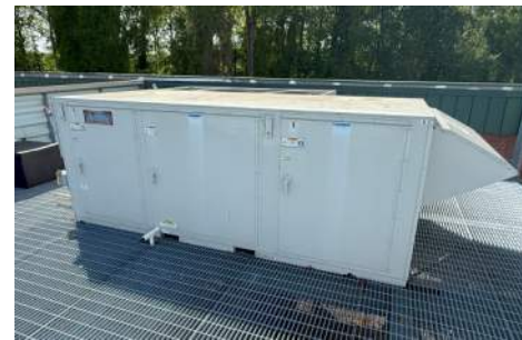
Existing Rooftop DOAS and Classroom Fan Coil Unit (Shown Above)
