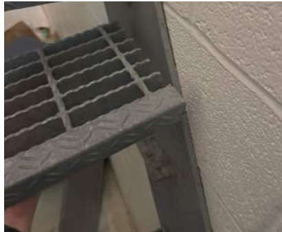
Figure 69 - Disconnected Tread
