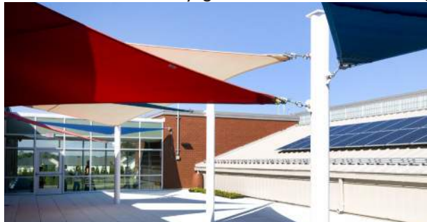
Outdoor Classroom on the roof with Wind Turbine
