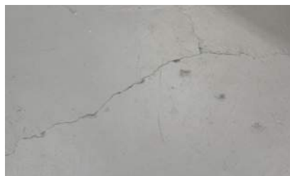
Figure 28 - Concrete Cracking
