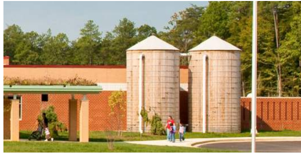
Green Roof and Cisterns for Storage Greywater
