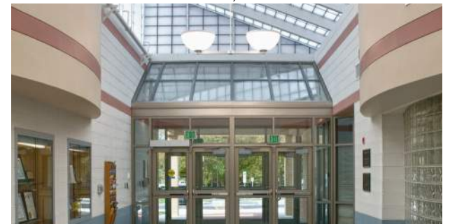
Natural Daylight at Secured Vestibule
