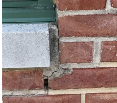
Figure 14 - Cracked Mortar
