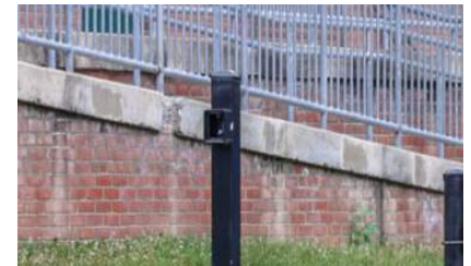
Figure 12 - Efflorescence
