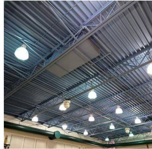
Existing Gymnasium and Exterior Metal Halide Luminaires
