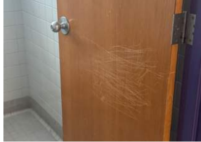
Figure 41 - Bathroom Wood Door
