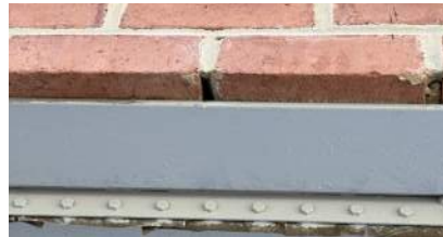
Figure 15 - Missing Mortar
