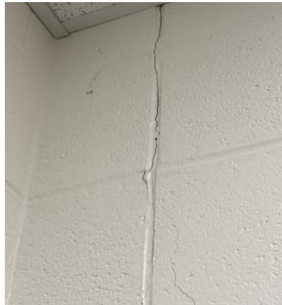
Figure 27 - CMU Cracking
