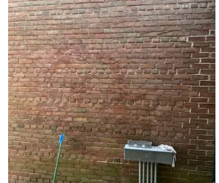
Figure 10 - Spalling Brick
