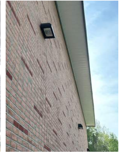
Existing Gymnasium and Exterior Metal Halide Luminaires
