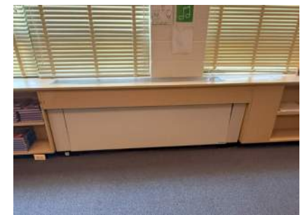
Existing Rooftop DOAS and Classroom Fan Coil Unit (Shown Above)
