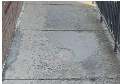
Figure 22 - Concrete Spalling
