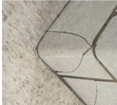
Figure 26 - GMU Cracking
