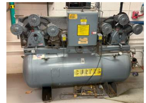
Existing Central Plant DDC Controller and Boiler Room Air Compressor
