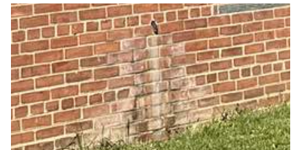
Figure 13 - Water damage
