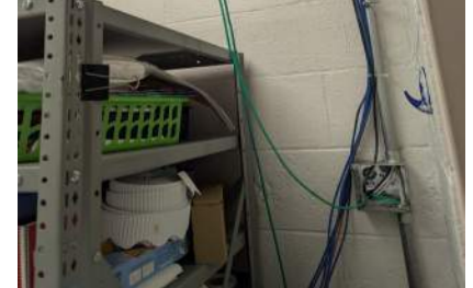
Figure 46 - Exposed Wiring
