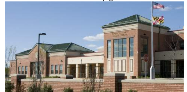
Access Control at the County's 1st Green Neighborhood
