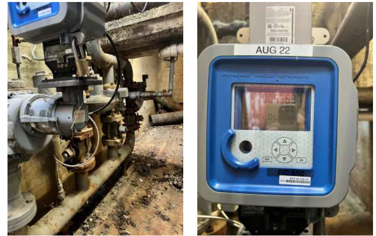
Existing Exterior Gas Service and Washington Gas Meter
