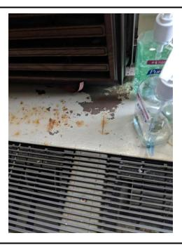
Photo 6: Deteriorated white paint on metal window sill (Negative XRF Readings)
