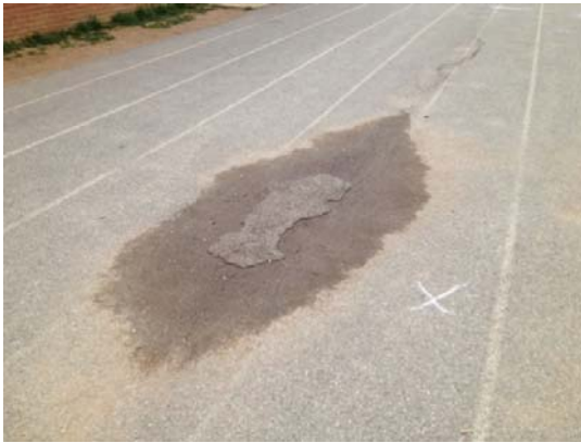
100 meter dash surface in poor on condition
