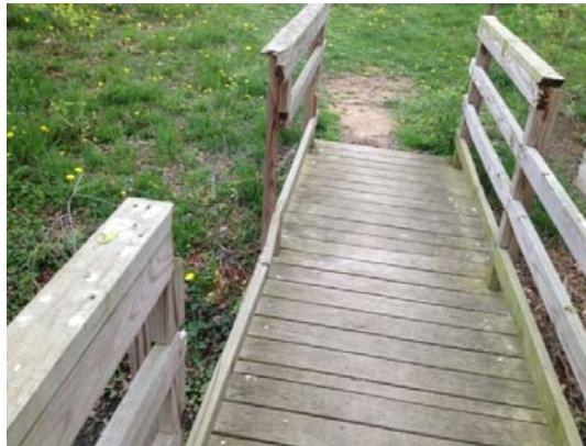
Unsafe pedestrian bridge
