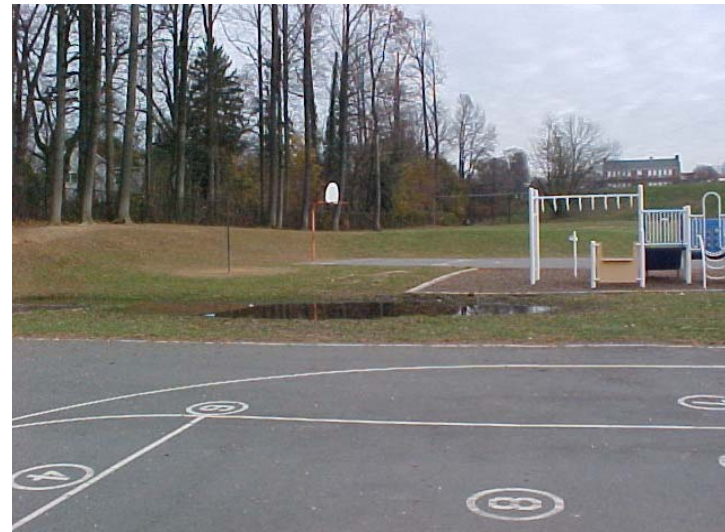
Ponding on grassy area
