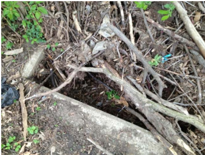
Clogged inlet location: west side of the parking lot
