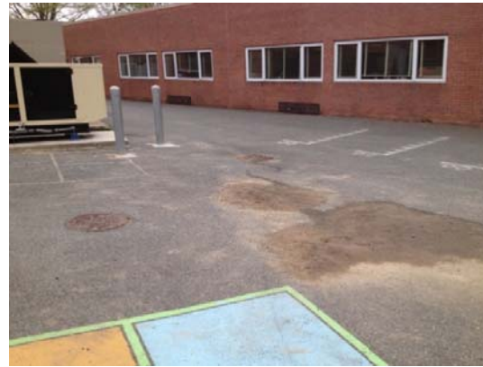
Ponding location: center hard play surface
