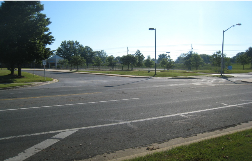
EXISTING BUS LOOP ENTRANCE
