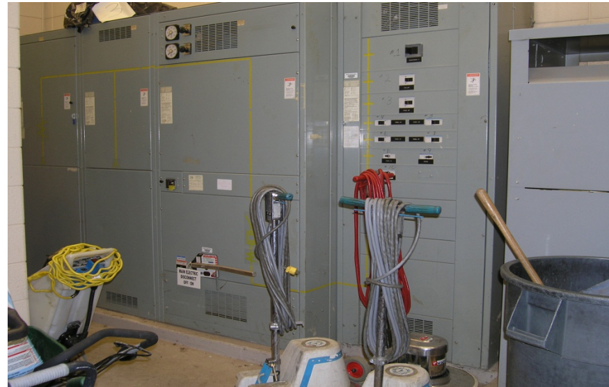
EXISTING ELECTRICAL SERVICE
