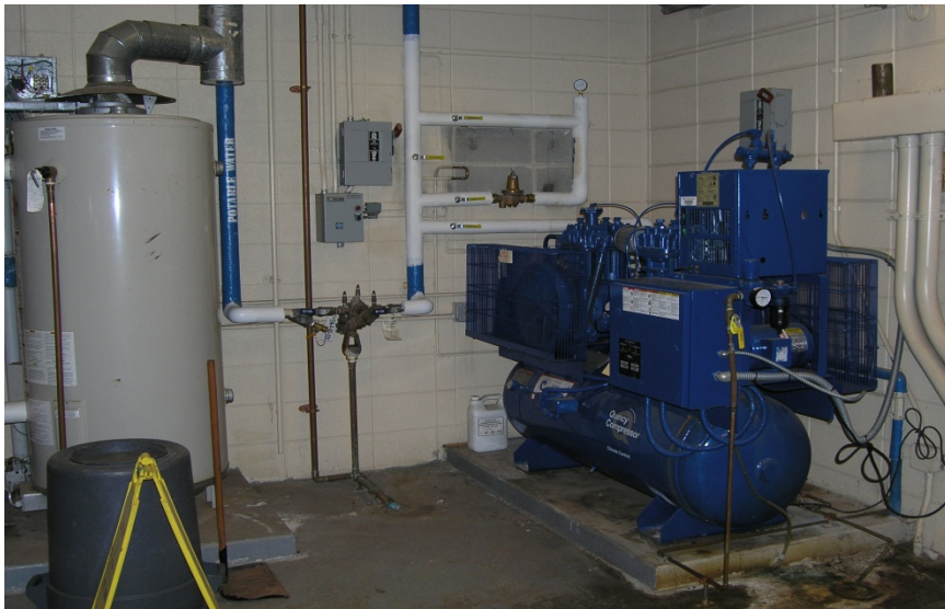
EXISTING WATER HEATER AND COMPRESSOR
