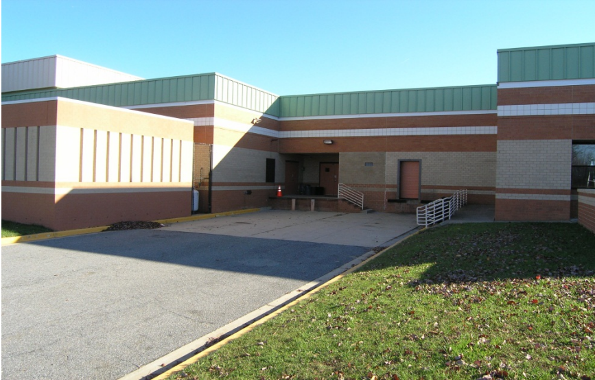
EXISTING LOADING DOCK
