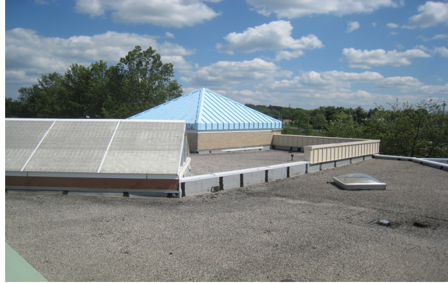
EXISTING ENTRY AND MEDIA ROOF
