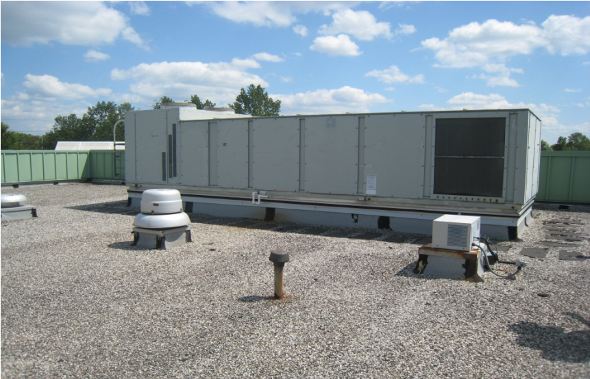
EXISTING ROOFTOP UNIT
