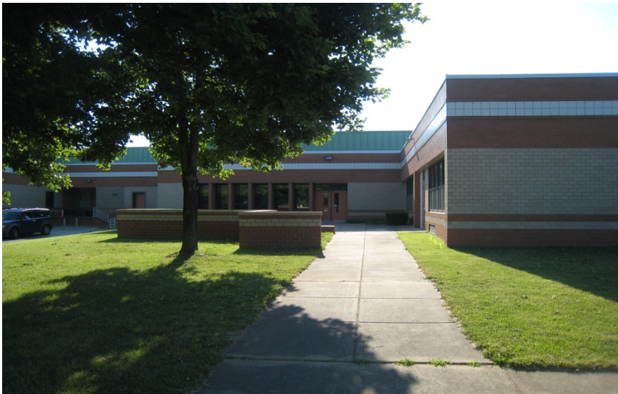
EXISTING ALL-PURPOSE ROOM ENTRY AND COURTYARD
