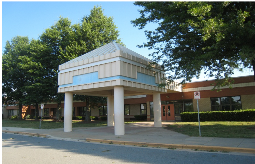
EXISTING DROP-OFF CANOPY
