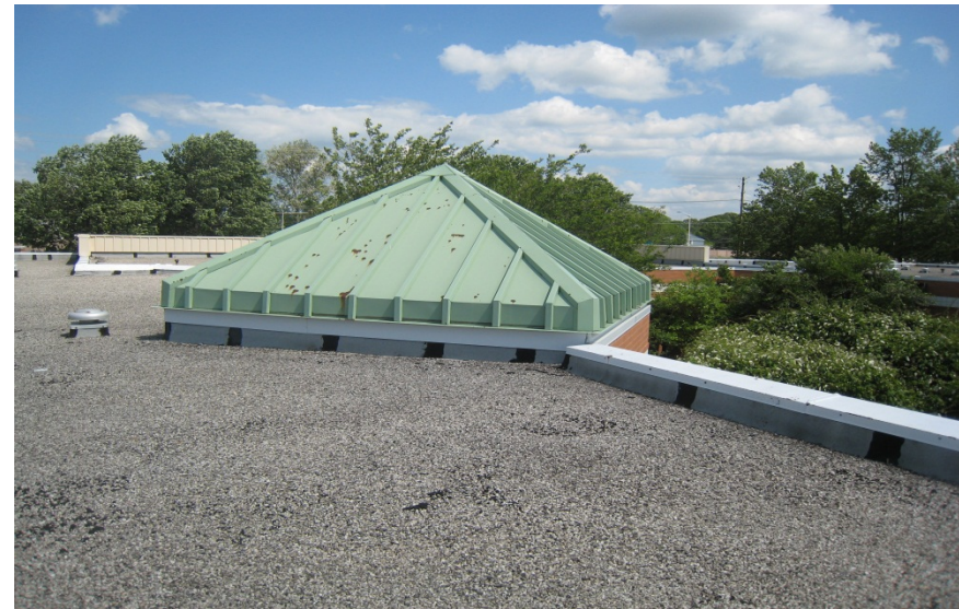
EXISTING STAFF LOUNGE ROOF FEATURE
