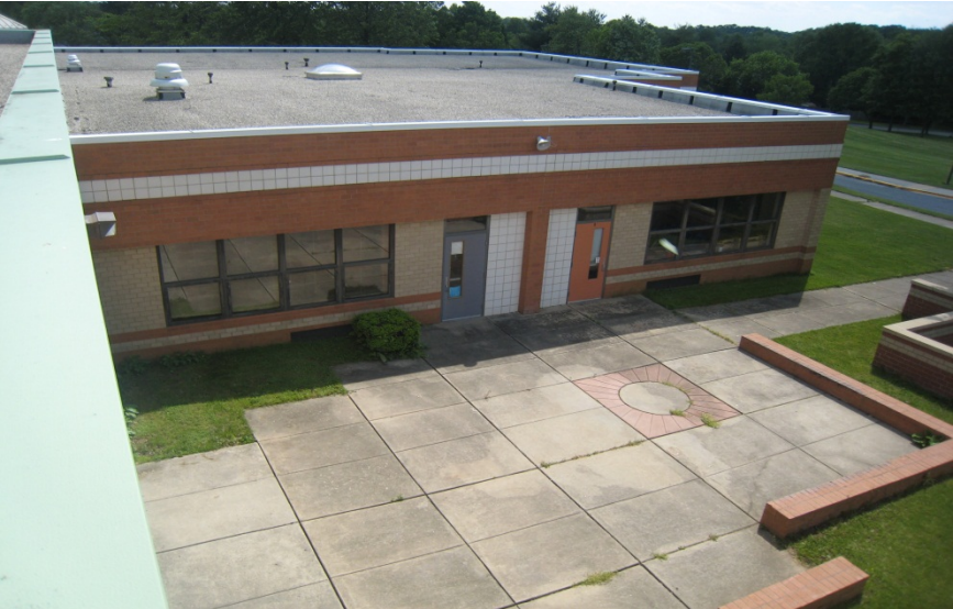
EXISTING ALL-PURPOSE ROOM/ART COURTYARD
