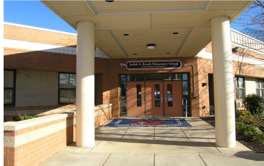
EXISTING MAIN ENTRY DOORS
