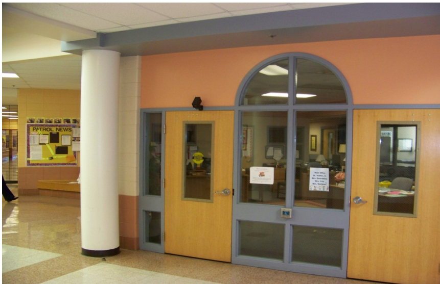
EXISTING MAIN OFFICE ENTRY
