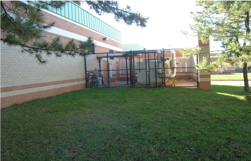
EXISTING CHILLER ENCLOSURE
