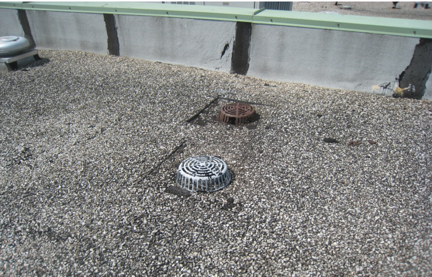
TYPICAL ROOF DRAIN
