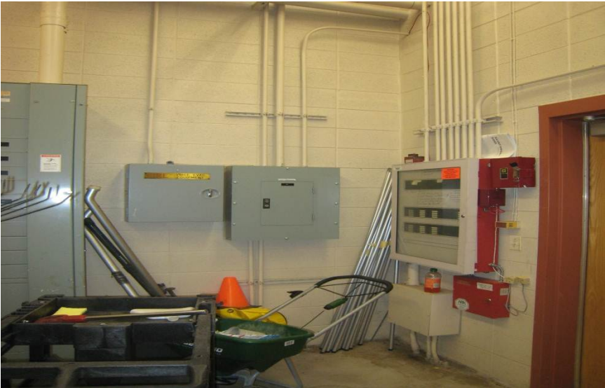
EXISTING ELECTRICAL ROOM
