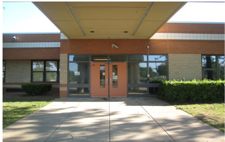
EXISTING DROP-OFF ENTRANCE
