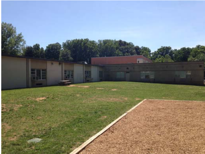
Site – North/West Façade from Play Area
