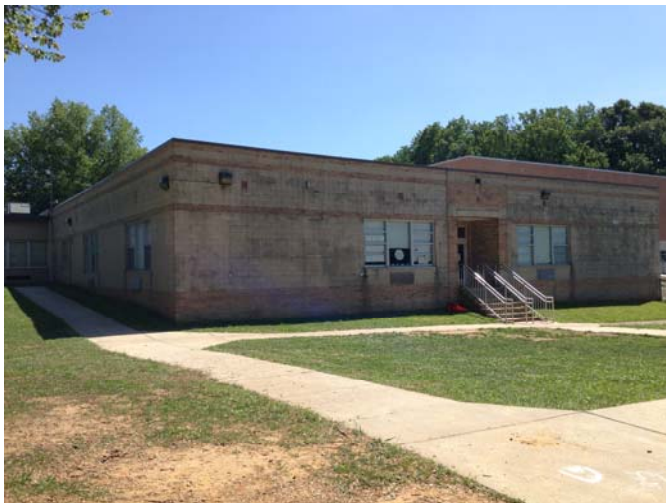
Site – 1988 Addition (North Façade)
