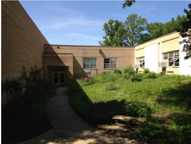
Site – 1988 Addition (South Façade)
