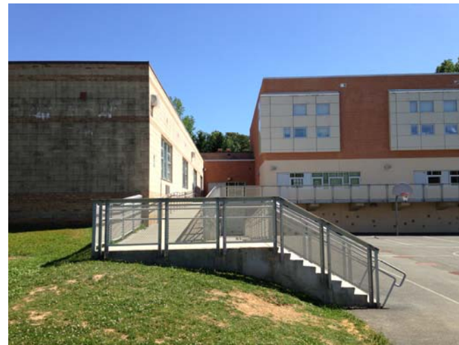
Site – 1988 & 2008 Addition (North Façade)
