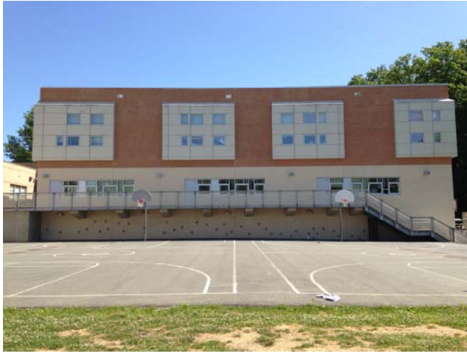
Site – 2008 Addition (North Façade)
