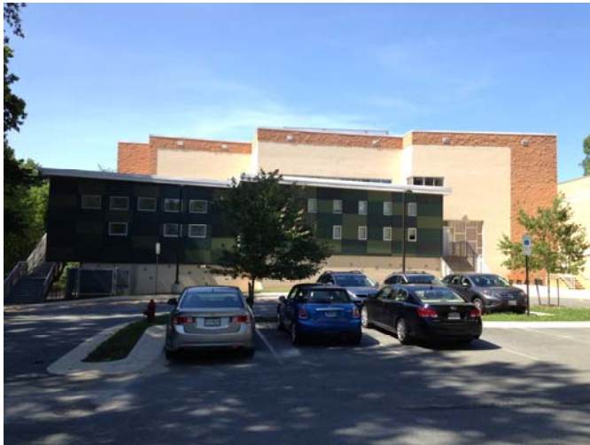
Site – 2008 Addition (South Façade)
