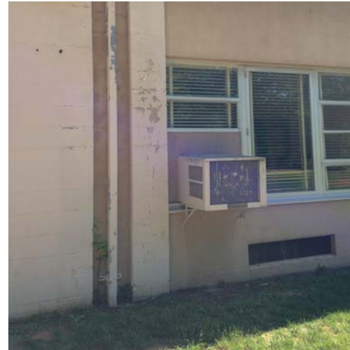
Site – Typical Classroom Window Opening
