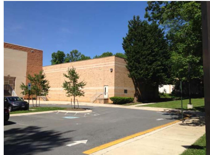
Site – 1988 Addition (Gymnasium Façade)
