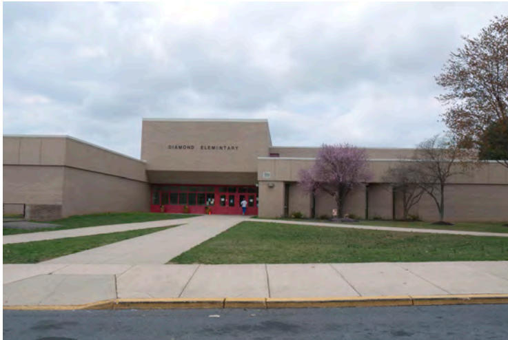
Front of building from bus loop
