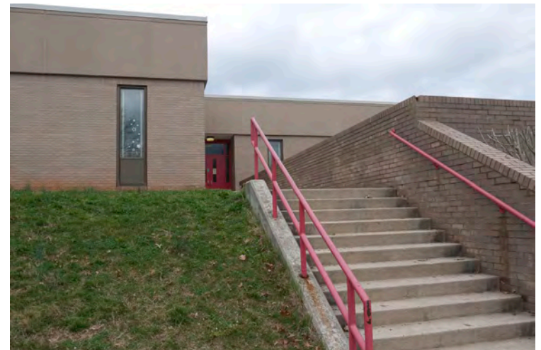
Stair from bus loop
