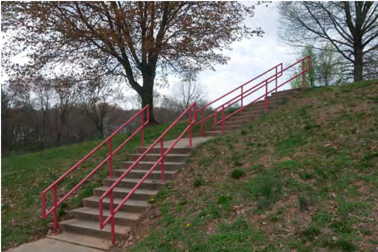
Stair from lower end of bus loop to playground
