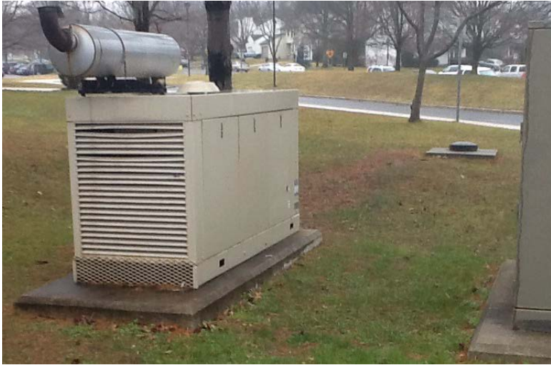
No screen wall around generator.
