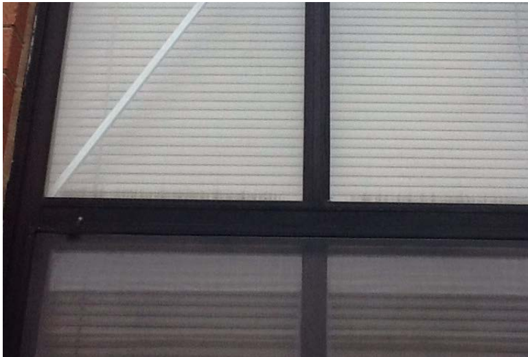
Window sash failure.
