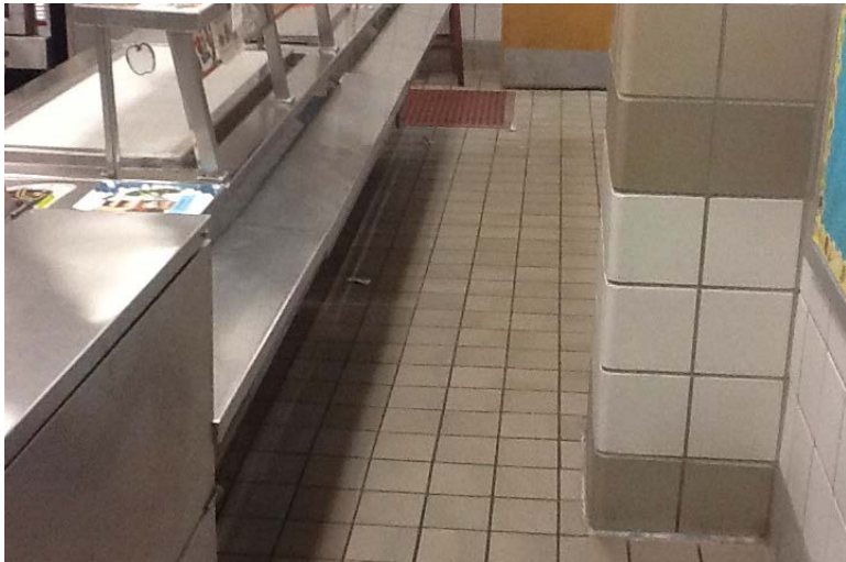
Kitchen's serving line is not ADA compliant due to existing column.
