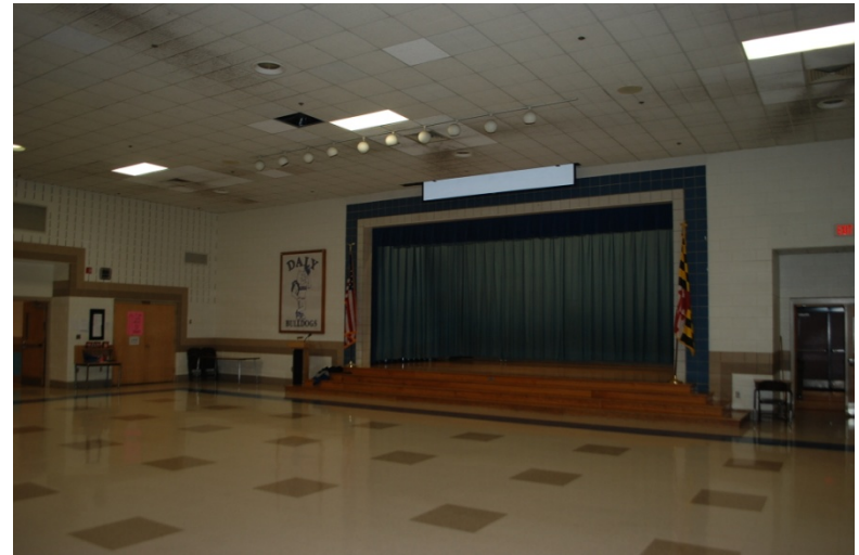
Multi - purpose room's ceiling excessively dirty.
