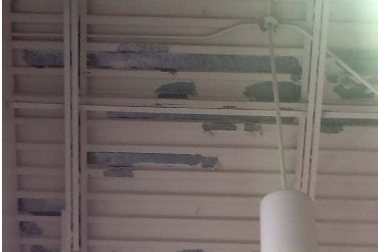
Vestibule ceiling's paint peeling.
