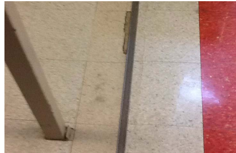
Floor is cracking and broken from settlement.
