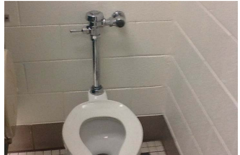
Bathrooms not ADA compliant.
