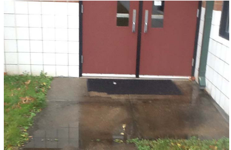
Roof drain spill onto egress sidewalks create icing hazard.
