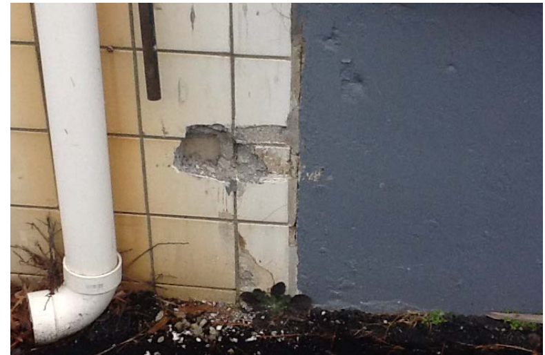
Minor damages to exterior wall.
