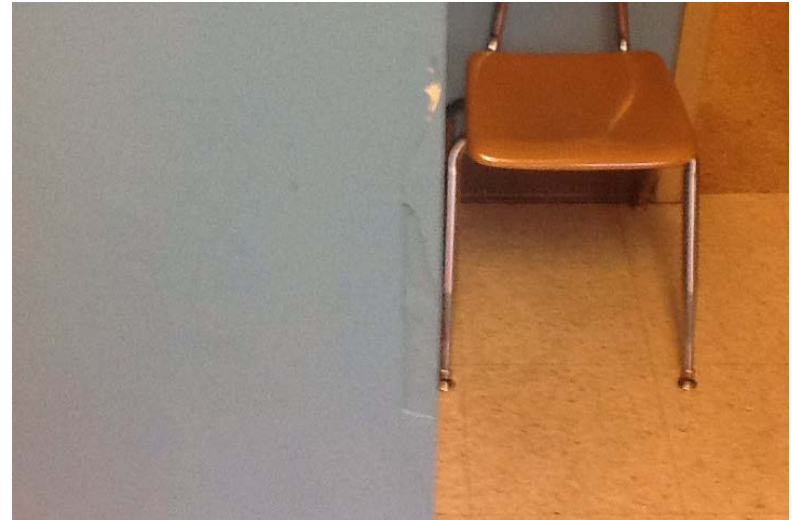
Minor damages to drywall within corridors.
