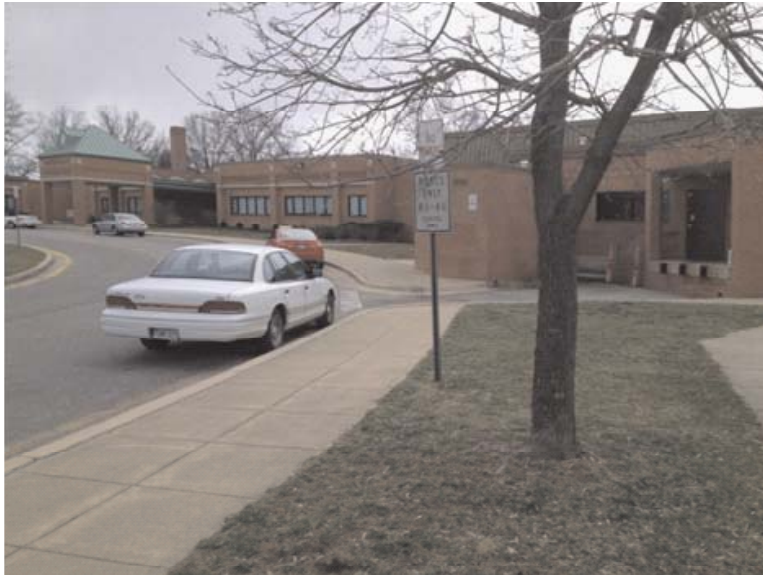
Front Entrance - Old Sidewalks Meet New
