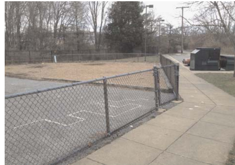
Front unused hard play surface and mulch area- from school facing south
