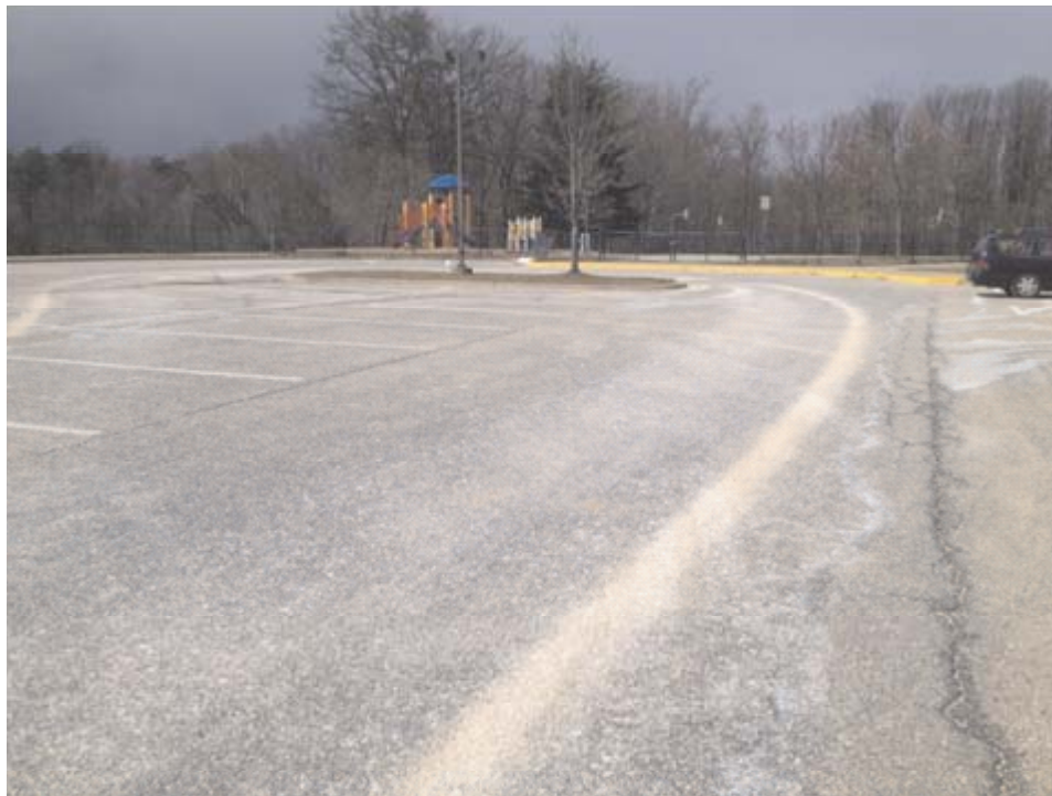
Side Parking Lot - Looking North at Student Drop-Off
