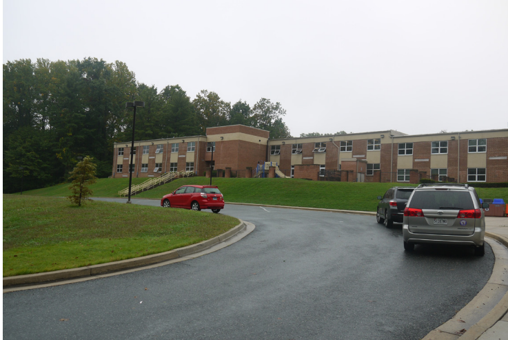
Front of building from bus loop
