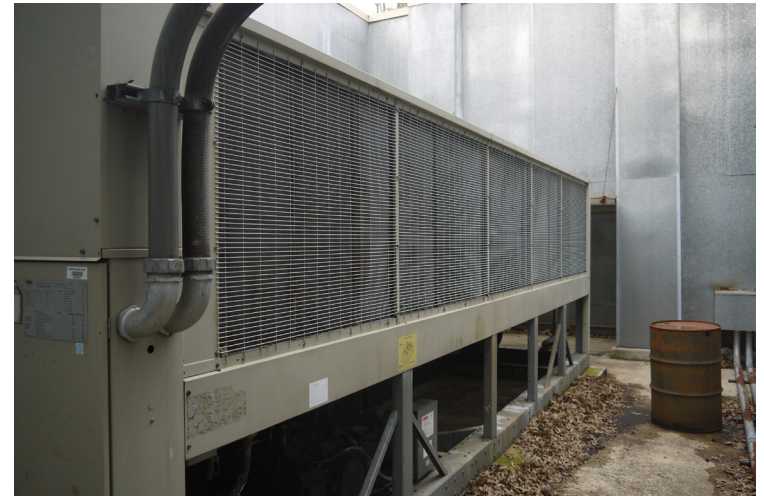
Outdoor air cooled condenser unit in sound lined enclosure
