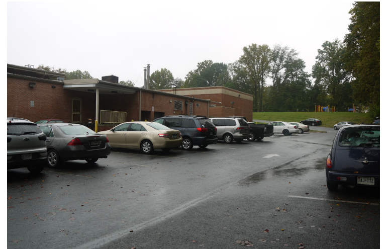
View of staff parking/loading area and student drop-off loop
