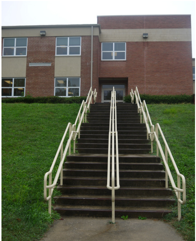
Stair from bus loop to classroom wing
