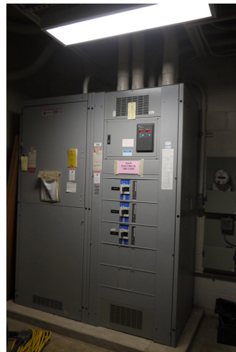
Main electrical panel
