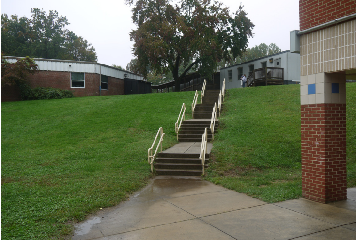
Stair from gymnasium to relocatables and play fields
