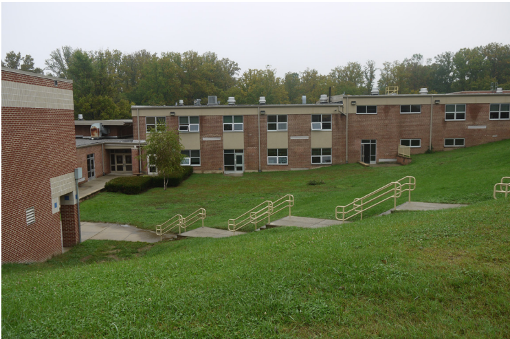
View looking toward classroom wing across terraced open space
