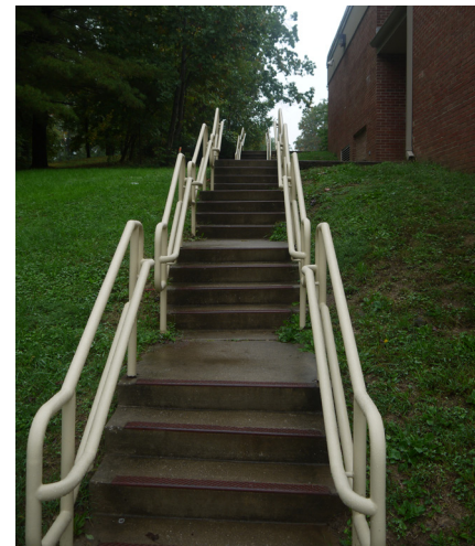
Stair at southeast end from bus loop
