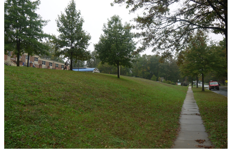
Embankment between bus loop and Nadine Drive
