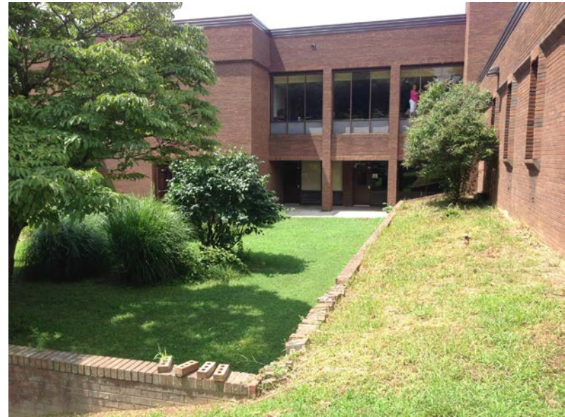
East Court Yard adjacent to the current Dining Room.
