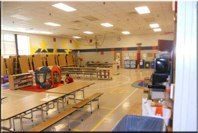
2B: Multipurpose Room - Interior
