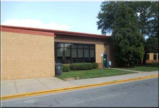
1B: Multipurpose Room - Exterior
