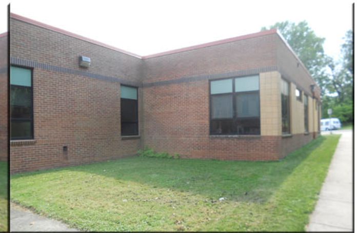
3B: Health Room - Exterior
