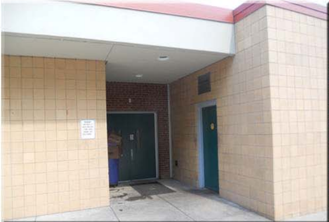
1C: Multipurpose Room - Exterior
