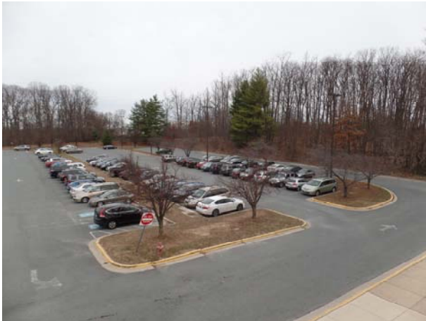
Figure F- Parking Lot
