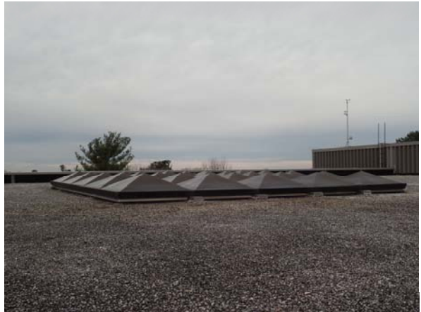
Figure H- Skylight above Ramp
